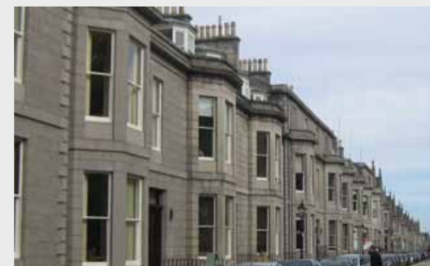
House with Sandstone Walling
