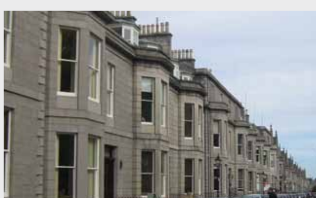
Rough Punched Balmoral Grey Granite Wall Coping Malmaison Hotel, Aberdeen Architect: Curious Architecture, Glasgow
