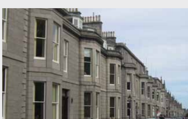
Rough Punched Balmoral Grey Granite Wall Coping Malmaison Hotel, Aberdeen Architect: Curious Architecture, Glasgow
