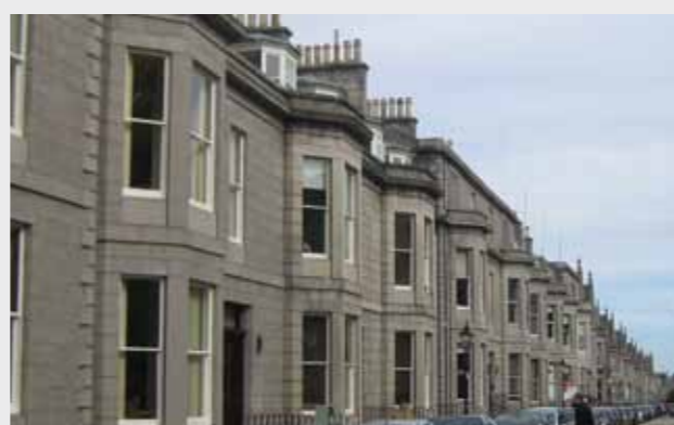
Rough Punched Balmoral Grey Granite Wall Coping Malmaison Hotel, Aberdeen Architect: Curious Architecture, Glasgow
