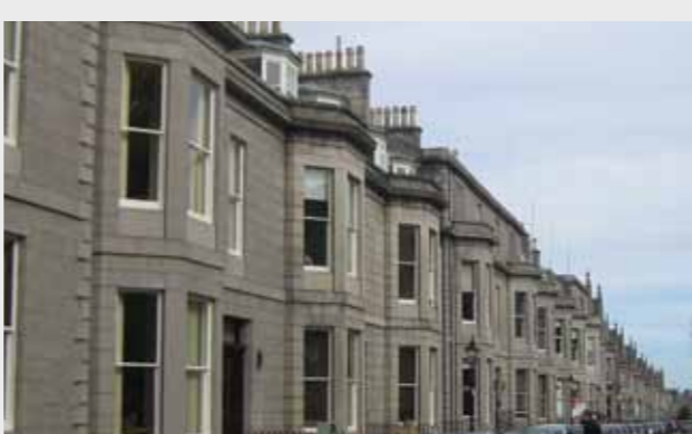
Rough Punched Balmoral Grey Granite Wall Coping Malmaison Hotel, Aberdeen Architect: Curious Architecture, Glasgow
